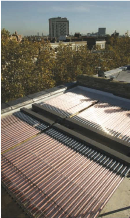
Solar water heating installation on the Flagship Home, London courtesy of the Royal Borough of Kensington and Chelsea
