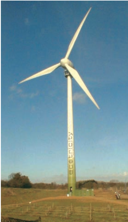
1.5 MW community wind turbine at the Ecotec Centre in Swaffham. Photo courtesy of Keith Richards, TVenergy.org
